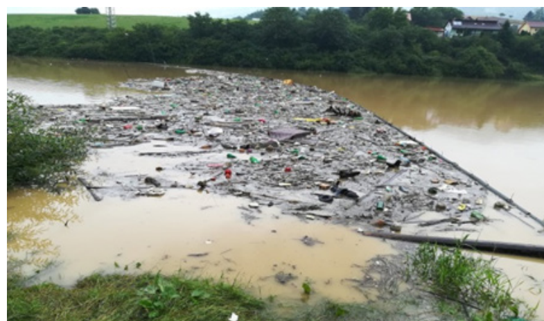
Figure 4. Waste captured with the use of a barrier wall in the area of the Ružín water reservoir
