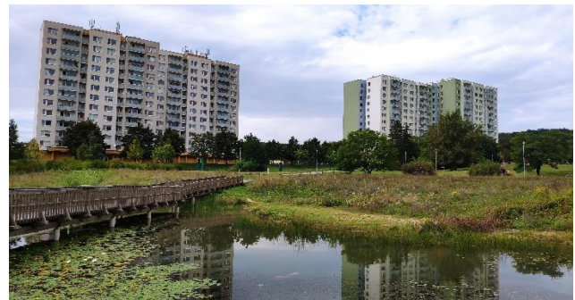
Figure 3. Above-ground retention tank in Brno, Czech Republic (source: Author, 2020)
