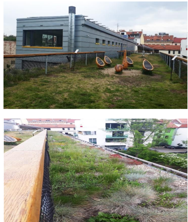
Figure 5. Green intensive roof at the passive building (source: Author, 2019)
